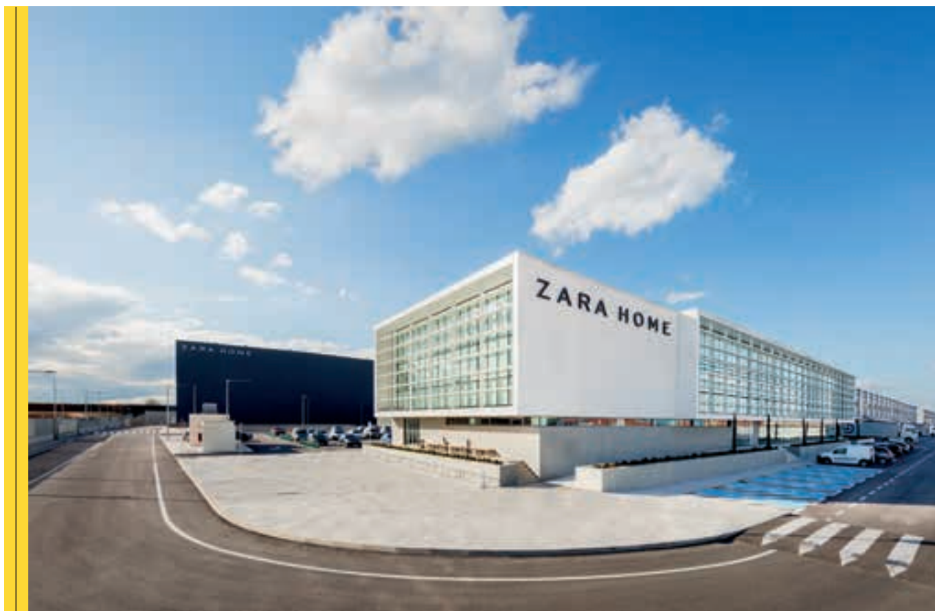
New Zara Home logistic premises in Cabanillas (Guadalajara), with LEED Gold certification.
